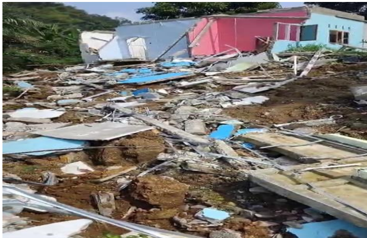
Figure 1 Destroyed resident's house
